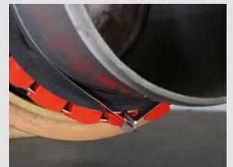
*Level-invert transitions: After pre-tensioning the clamping screws, the T-socket wrench is applied to the set screw on the top (arrow) to bring the components to invert-level. This also ensures the absorption of shear forces, thanks to the design. Please note the detailed installation instructions enclosed with the BSM adaptor.*
